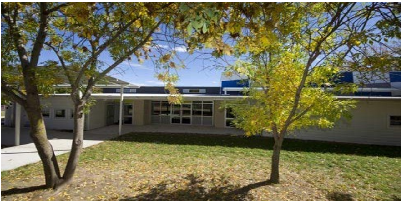
Figure 1: Front entrance to Torrens Primary School
